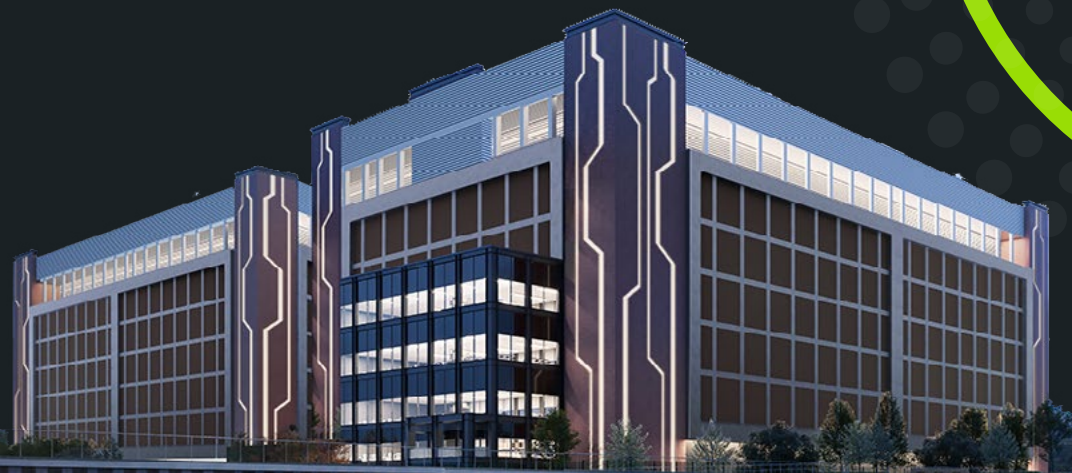
DOCKLANDS DATA CENTRE CAMPUS FROM THE RIVER THAMES
